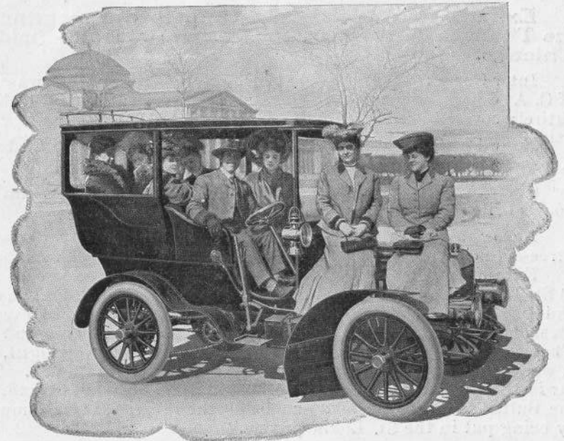
NO LOAD TOO MUCH FOR THE THOMAS.
