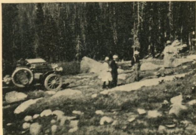
WORSE THAN NO ROAD AT ALL
