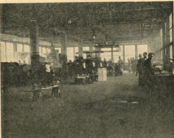
FINAL ASSEMBLING DEPARTMENT
