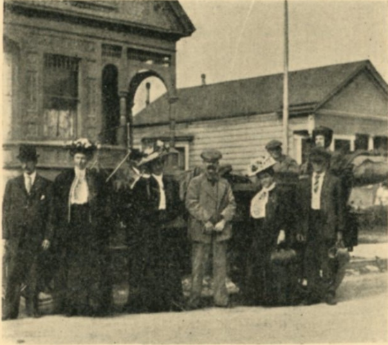
LEAVING OAKLAND, CAL., MAY 20, 1909
