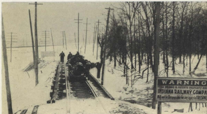
Between Goshen and South Bend over a trestle
