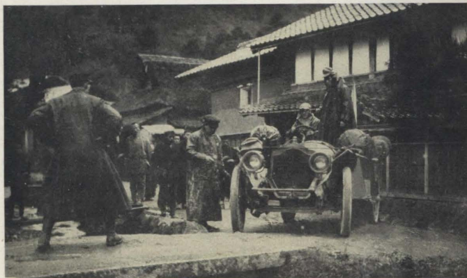
Maneuvering to cross narrow bridge
